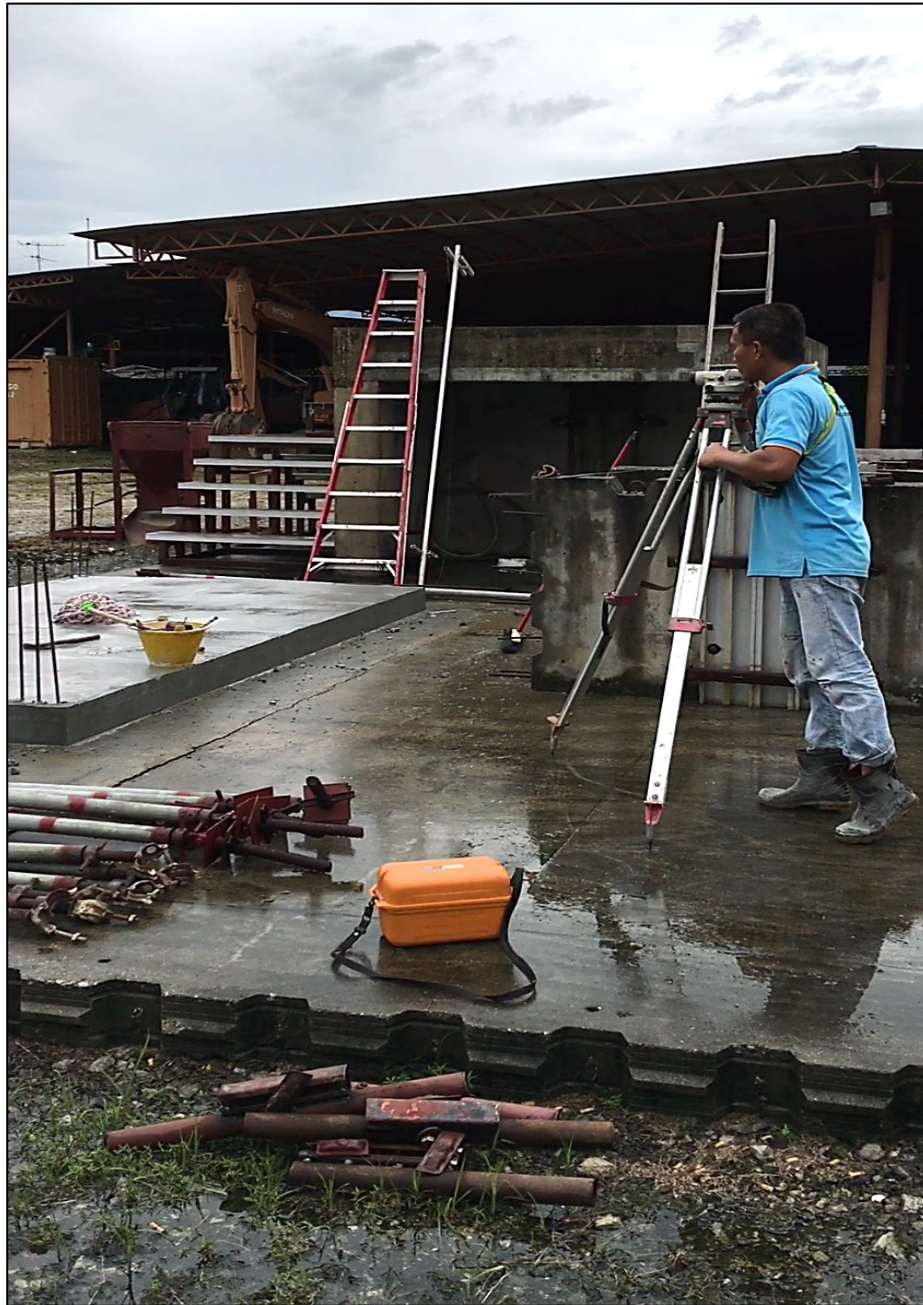
12 th & 13 th August 2018 : - Setting-out for panel installation
