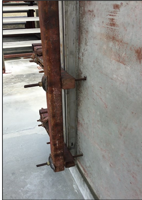
12 th & 13 th August 2018 : - Mock up panel wet joint ready for casting (on-site)
