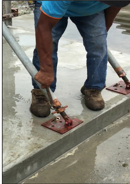
12 th & 13 th August 2018 : - Mock up panel wall prop dismantle (on-site)
