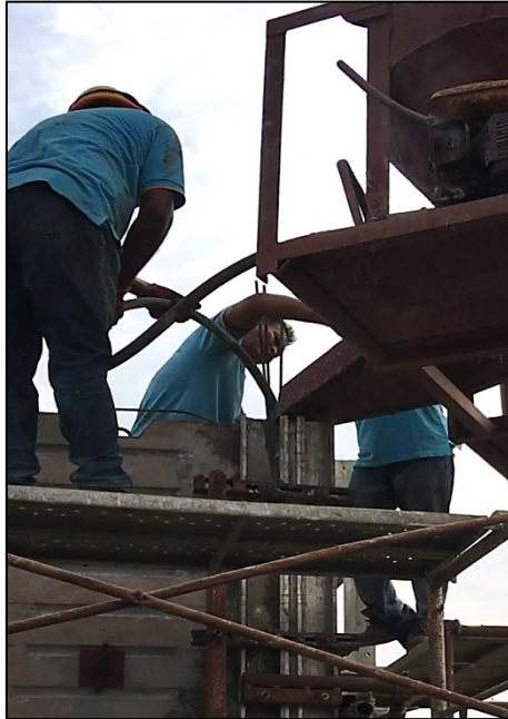
12 th & 13 th August 2018 : - Mock up panel wet joint casting (on-site)
