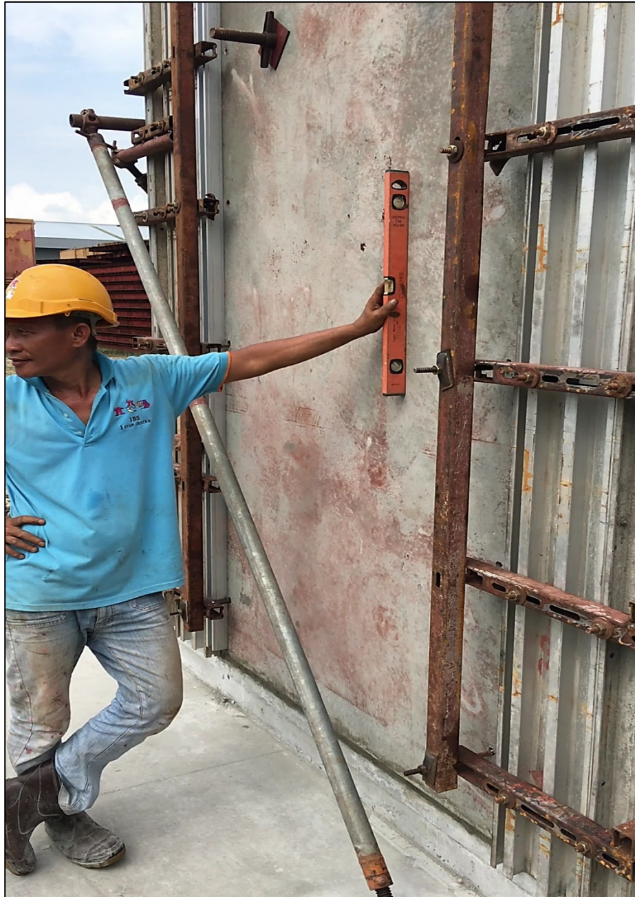
12 th & 13 th August 2018 : - Mock up panel Verticality checking before casting (on-site)
