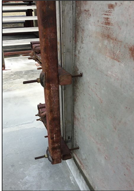
12 th & 13 th August 2018 : - Mock up panel wet joint ready for casting (on-site)
