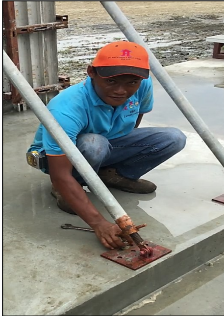
12 th & 13 th August 2018 : - Mock up panel wall prop dismantle (on-site)
