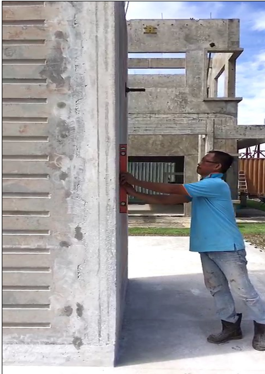
12 th & 13 th August 2018 : - Mock up panel Verticality (on-site)
