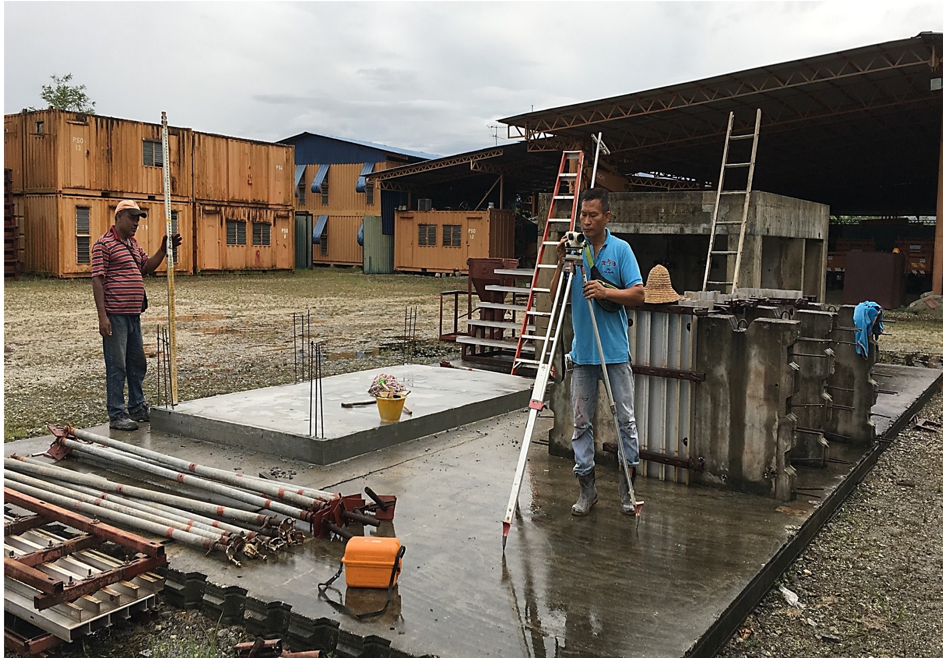
12 th & 13 th August 2018 : - Setting-out for panel installation
