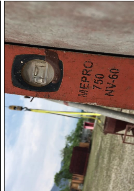
12 th & 13 th August 2018 : - Mock up panel Verticality checking before casting (on-site)
