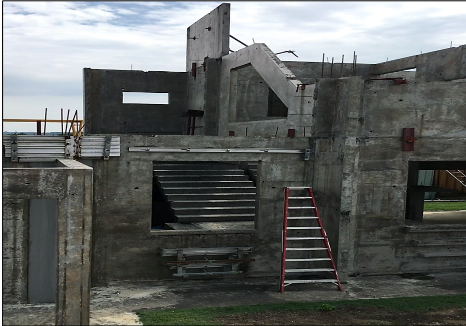
12 th & 13 th August 2018 : - Mock up panel wet joint ready for casting (on-site)
