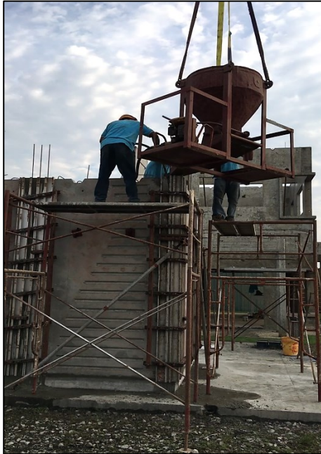
12 th & 13 th August 2018 : - Mock up panel wet joint casting (on-site)
