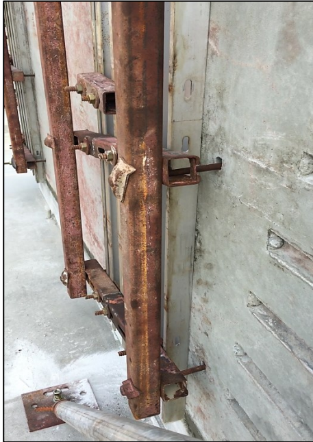
12 th & 13 th August 2018 : - Mock up panel wet joint ready for casting (on-site)
