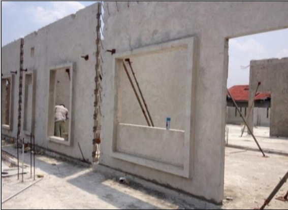
Load bearing wall
