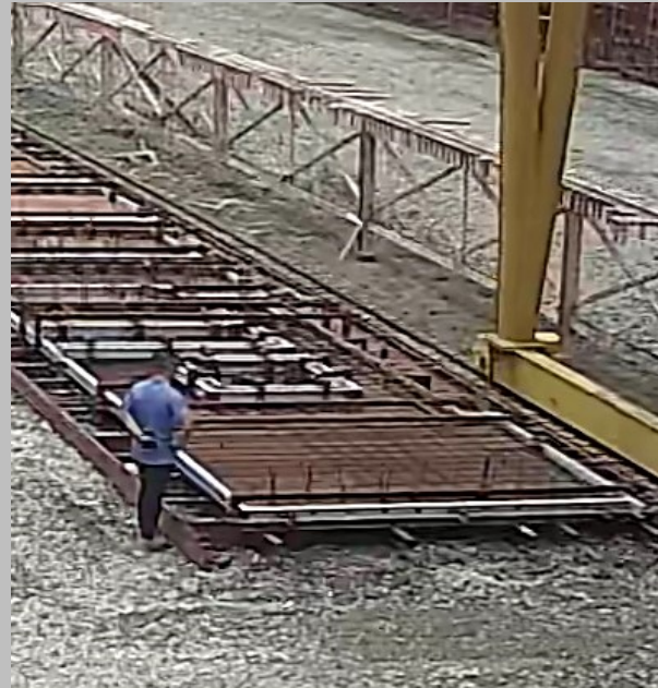
- 25 th Sept 2019 : Production yard - Precast panel wall casting sequence
