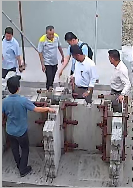
- 23 rd July 2019 Mock-up panel : Discussion on monolithic wall system with modular shear key (wet joint)
