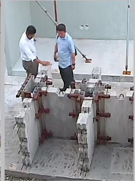
- 23 rd July 2019 Mock-up panel : Inspection on monolithic wall system with modular shear key (wet joint)
