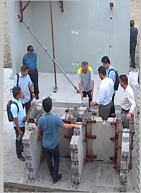
- 23 rd July 2019 Mock-up panel : Discussion on monolithic wall system with modular shear key (wet joint)
