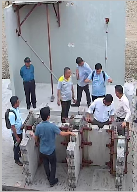
- 23 rd July 2019 Mock-up panel : Discussion on monolithic wall system with modular shear key (wet joint)
