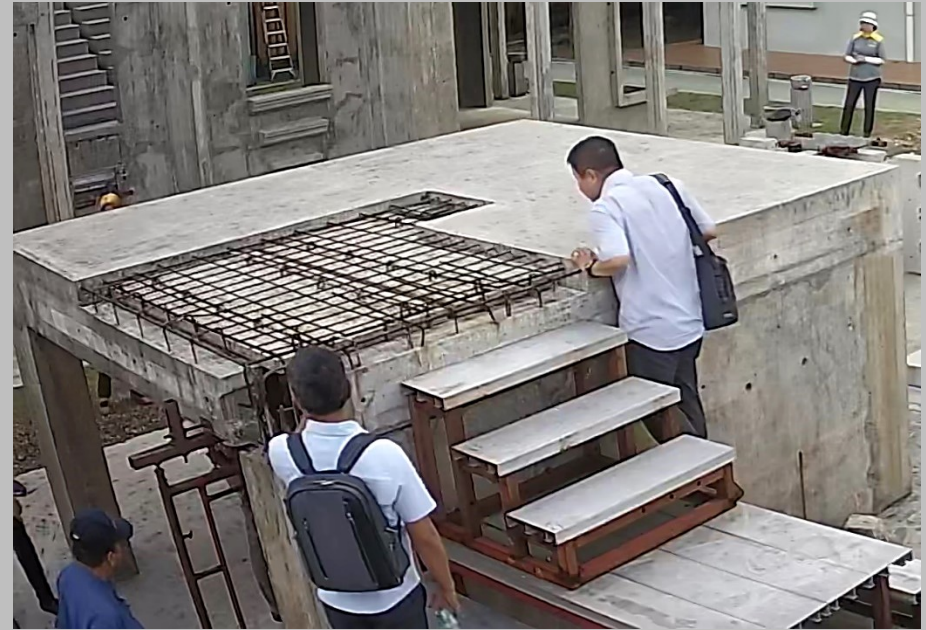
- 23 rd July 2019 Half slab sample unit : HC Precast Half slab with in-situ topping
