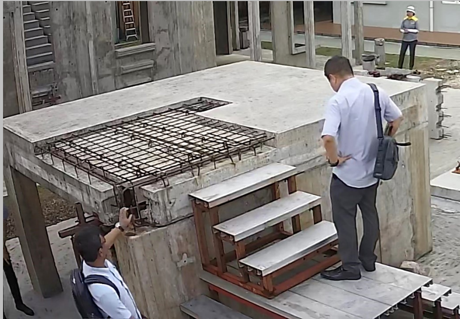
- 23 rd July 2019 Half slab sample unit : HC Precast Half slab with in-situ topping
