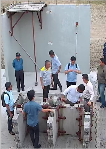
- 23 rd July 2019 Mock-up panel : Discussion on monolithic wall system with modular shear key (wet joint)
