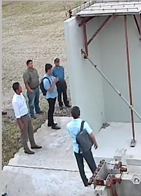
- 23 rd July 2019 Mock-up panel : Inspection on monolithic wall system with modular shear key (wet joint)
