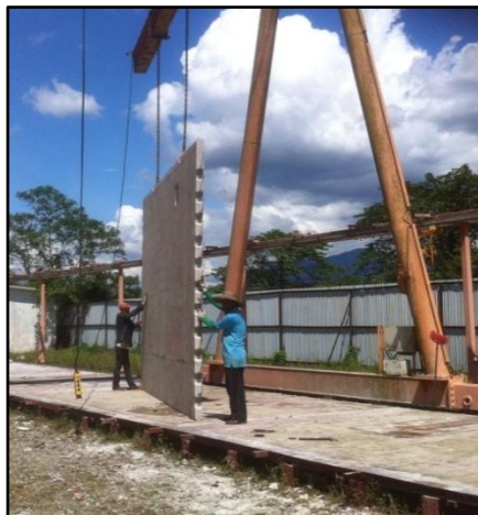
Panel 18 hrs hoist
