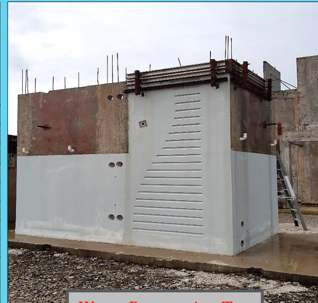
Water Penetration Test
