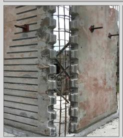
few one-stop precast system provider in which not only we own the earthquake resistant monolithic wall with multi-box system with key features of the connecting shear keys that possess tested structural integrity and preventing water leakage in wet climate environment as well as eliminating the possibility of zigzag crack along the connecting zone
