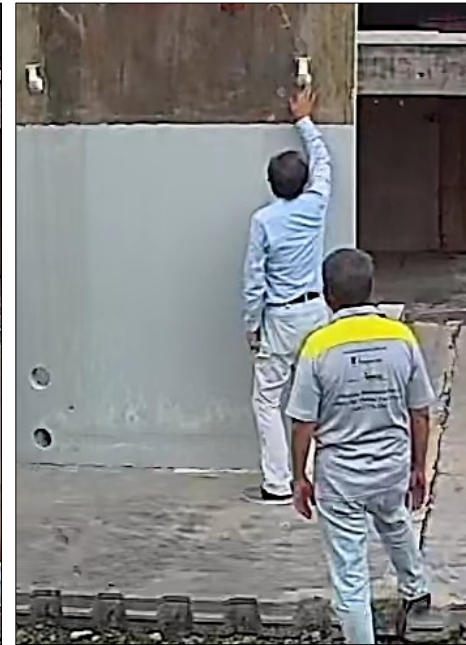
16 th November 2019 (After 24 hours) : - Inspection of Any Leaking Before Taking Water Level Reading
