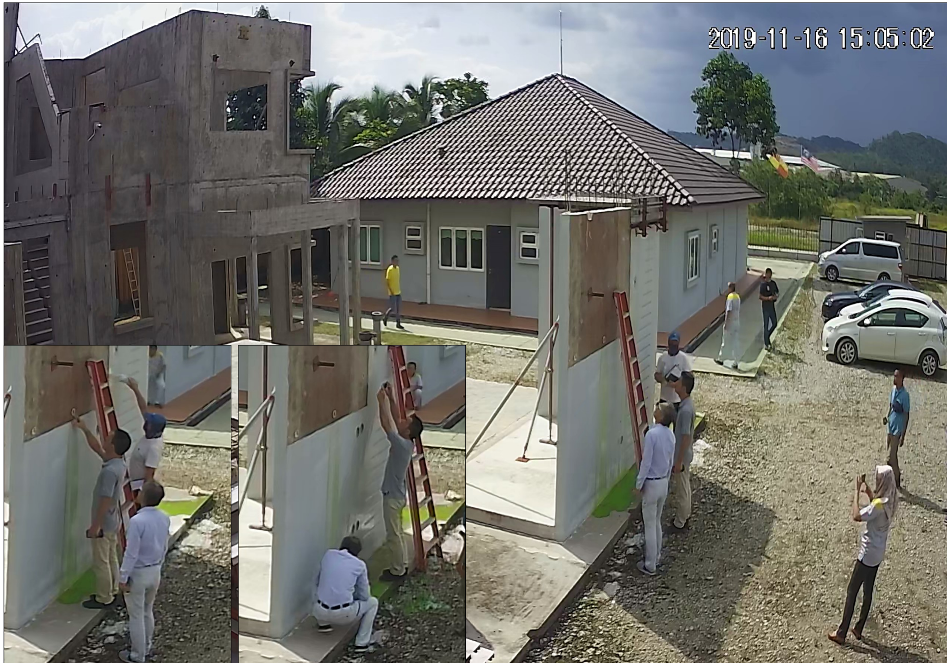
16 th November 2019 (After 24 hours) : - Inspection on HCPS's Modular Shear Keys to avoid leaking & cracks
