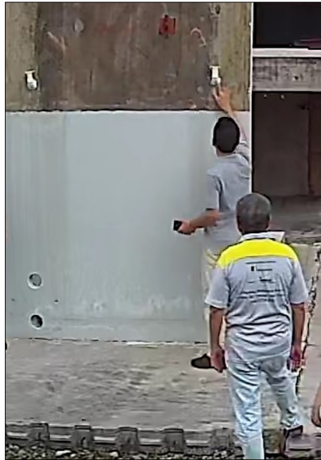
16 th November 2019 (After 24 hours) : - Inspection of Any Leaking Before Taking Water Level Reading
