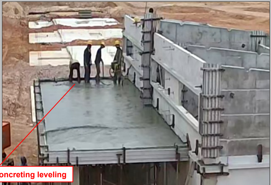
- In-situ flat roof concreting leveling
