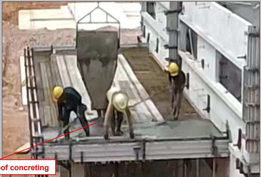
- In-situ flat roof concreting
