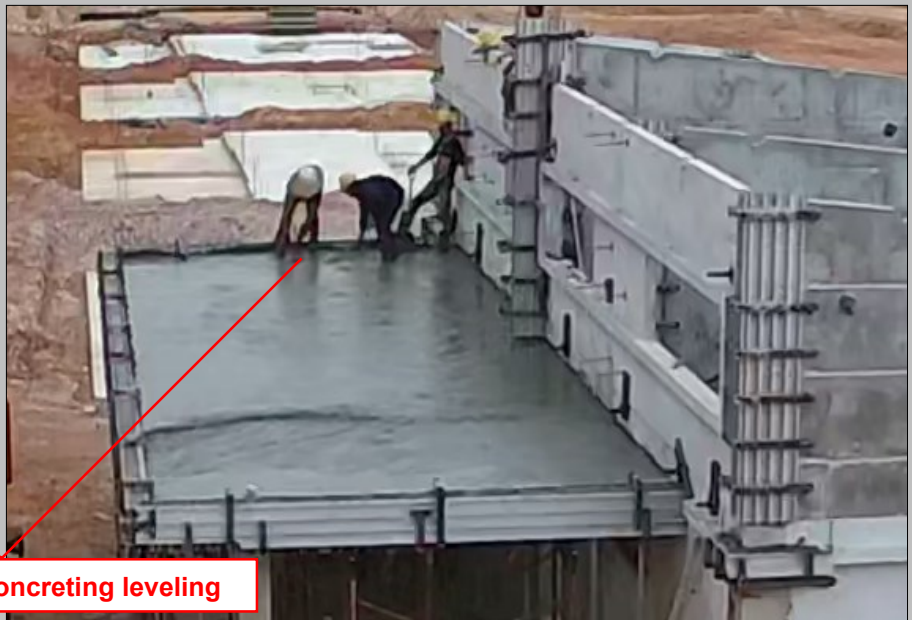
- In-situ flat roof concreting leveling
