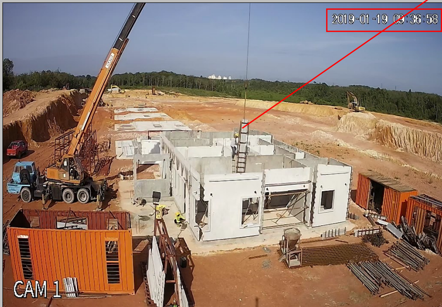
- Wet joint modular mould installation
