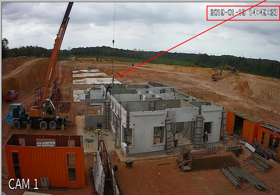
- Wet joint modular mould installation
