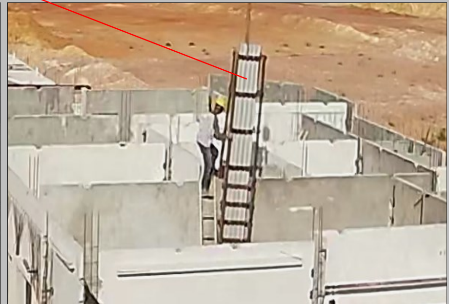
- Wet joint modular mould installation
