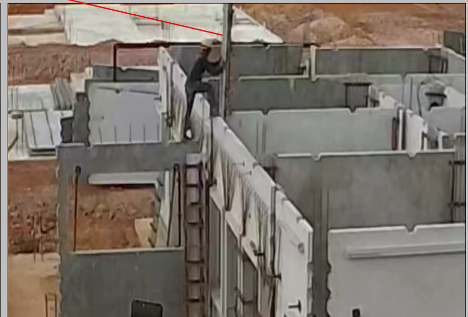
- Wet joint modular mould installation
