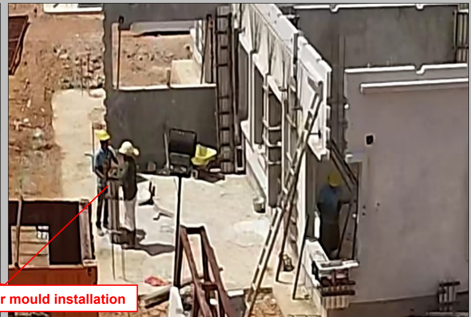
- Wet joint modular mould installation
