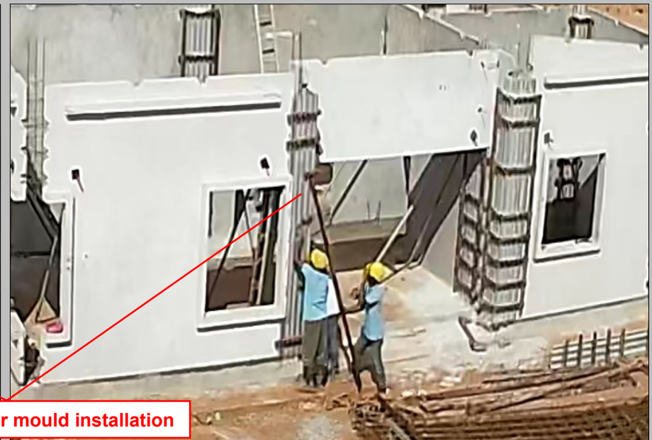
- Wet joint modular mould installation
