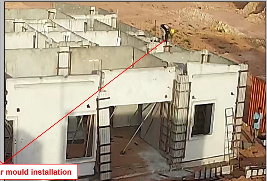
- Wet joint modular mould installation
