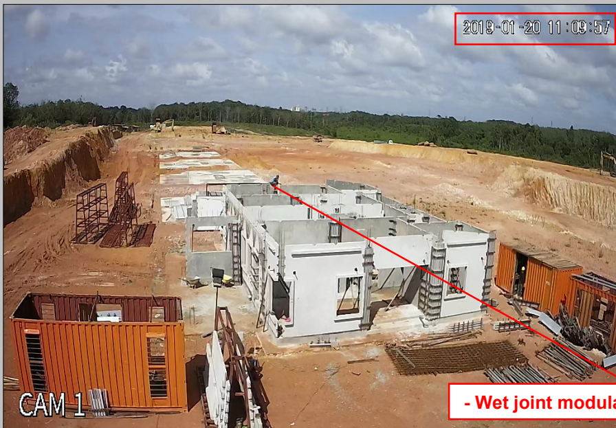
- Wet joint modular mould installation
