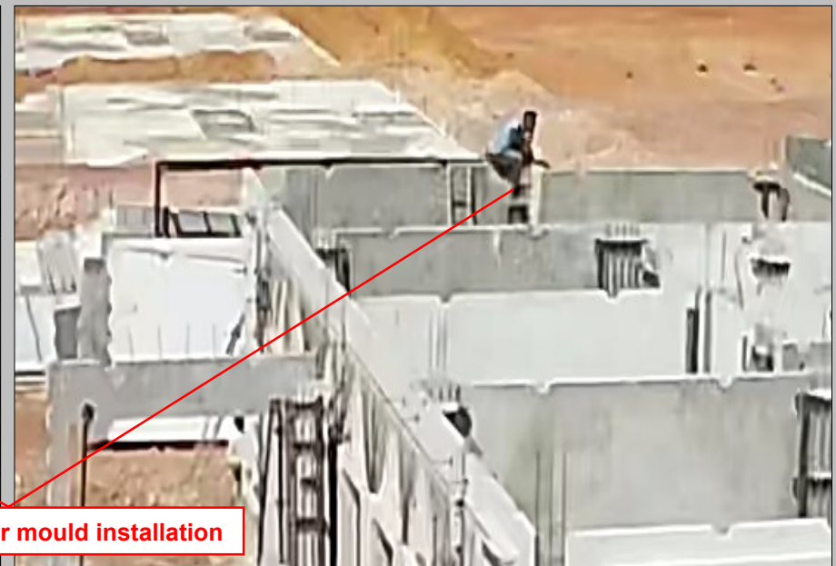
- Wet joint modular mould installation
