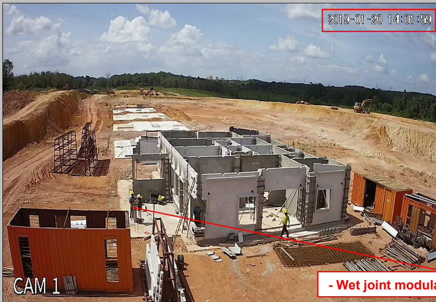
- Wet joint modular mould installation
