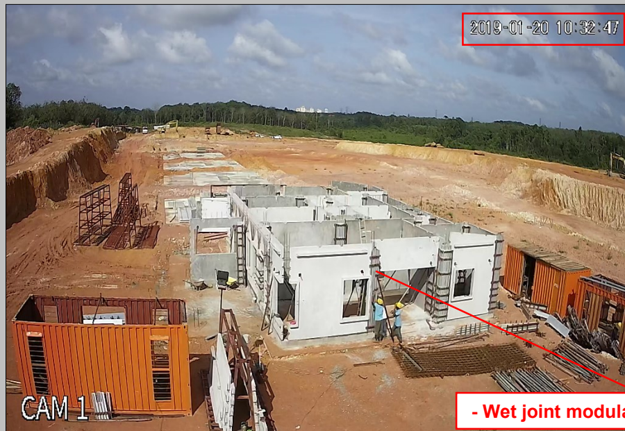
- Wet joint modular mould installation
