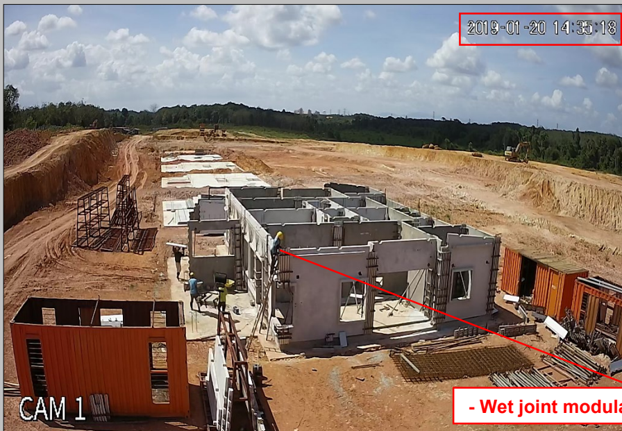
- Wet joint modular mould installation
