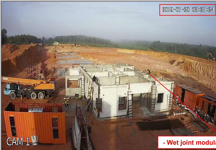
- Wet joint modular mould installation
