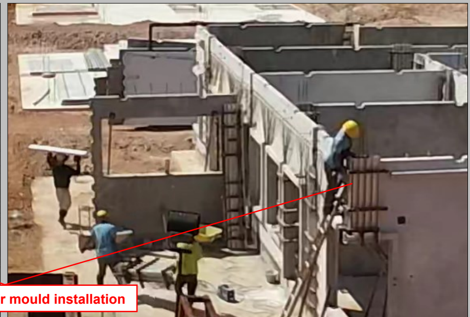
- Wet joint modular mould installation
