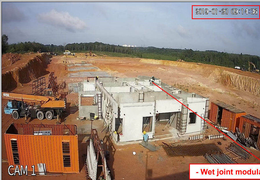
- Wet joint modular mould installation
