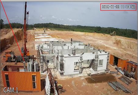
6. Day 5 ( 22/01/2019 ) : - Precast half slab & In-situ modular mould installation for flat roof at water tank area
